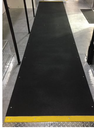
Panel installed on walkway
