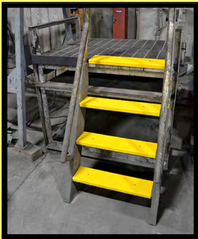
Fiber Glass Step Covers Interior Installation
